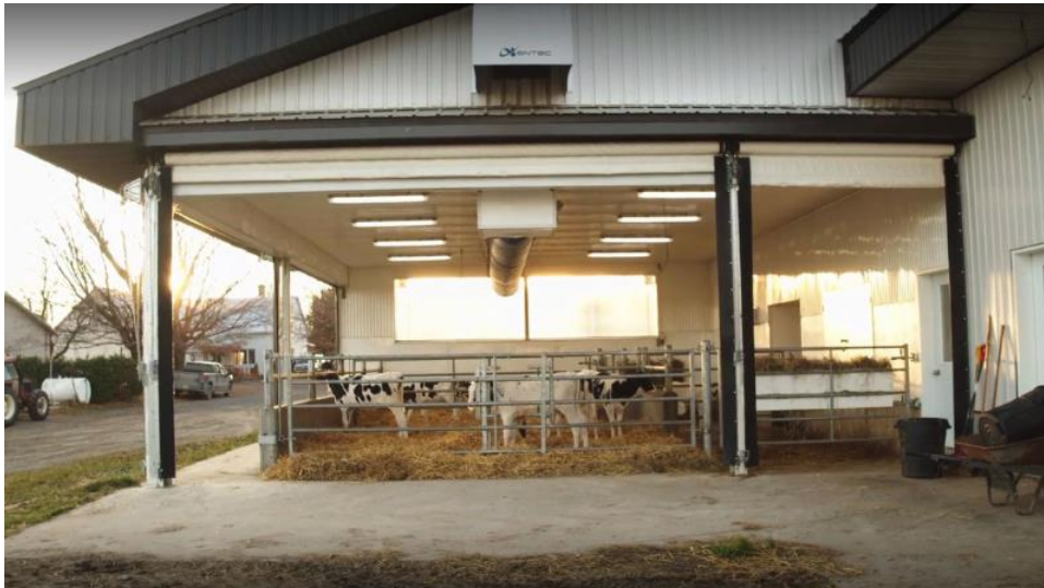
Figure 6: Example of group-housed calves with natural ventilation option, Source: Ferme Karona
