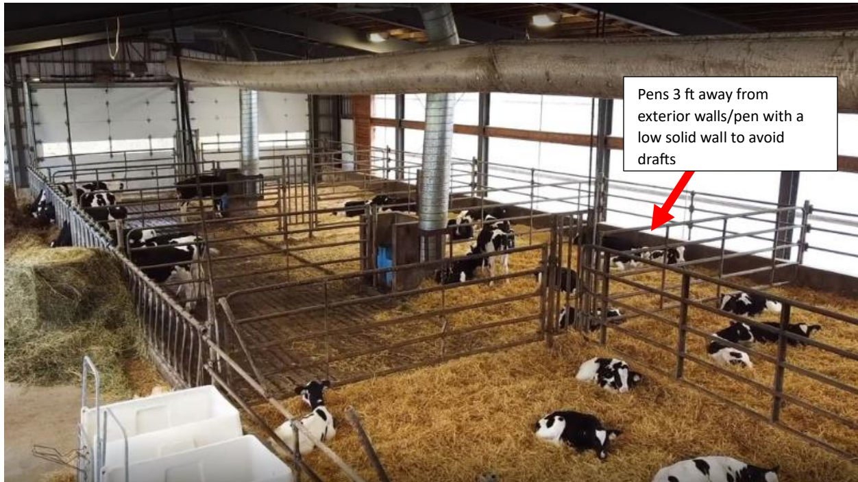
Figure 10: Natural ventilation with positive pressure ventilation, Source: Ferme Mystique S.E.N.C.
