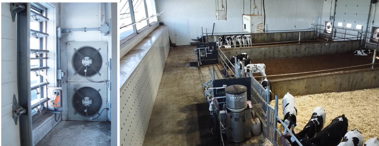
Figure 9. Separate calf building using fans to pull fresh air into the building and distribute evenly through the building via perforated walls, using exhaust fans to direct air towards the calf area and expel air out of the barn (neutral pressure ventilation). Additional air inlets can be seen above the perforated wall to increase the flow of fresh air in the summer, Source: Ferme Belvallée Inc.
