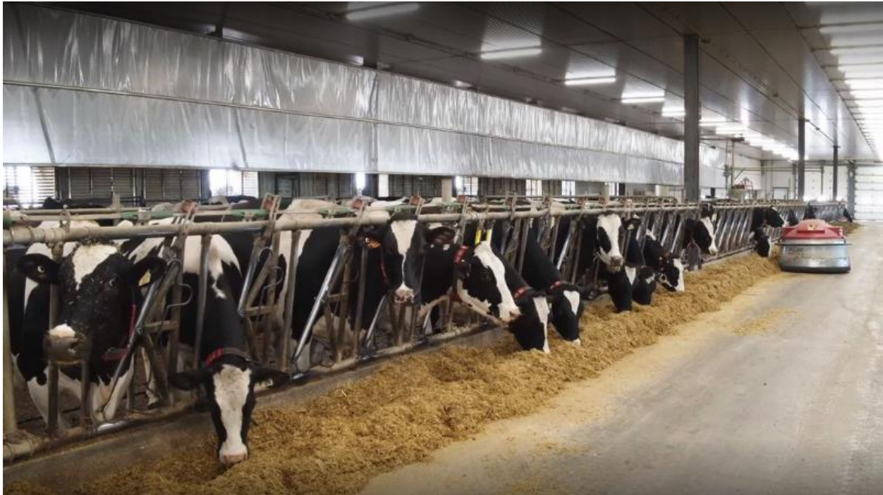
Figure 3: Baffles positioned over dairy cow resting area in cross ventilation barn, Source: Ferme Belvallée inc.
