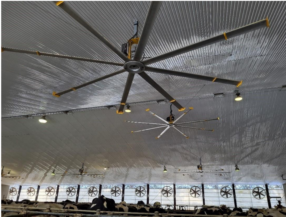
Figure 8. High volume low speed (HVLS) recirculation fans positioned on barn ceiling, Source: Ferme Caribou
