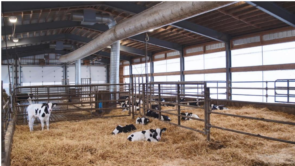
Figure 5. Positive pressure air tube ventilation system in a calf barn supplementing a natural ventilation system, Source: Ferme Mystique S.E.N.C.
