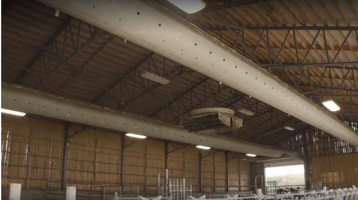
Figure 4. Positive pressure air tube ventilation system used to supplement air flow in the building, Source: Ferme Laperle inc.
